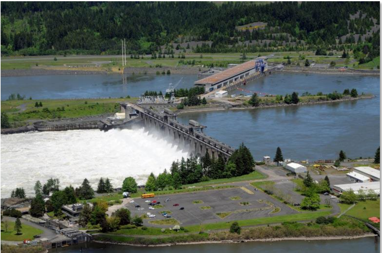
Spill at Bonneville Dam
