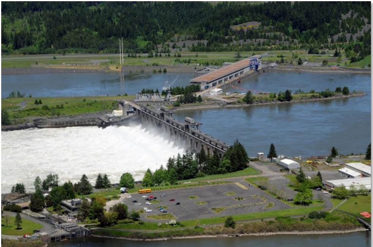
Spill at Bonneville Dam
