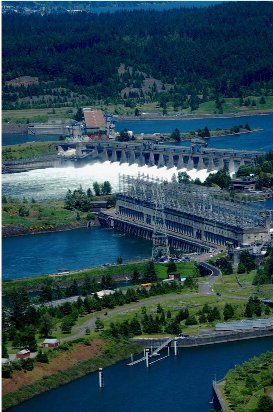
Bonneville Dam (Photo courtesy of Dennis Schwartz)
