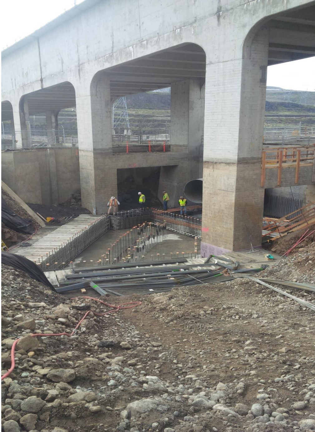
Concrete placement for 7' valve room.
