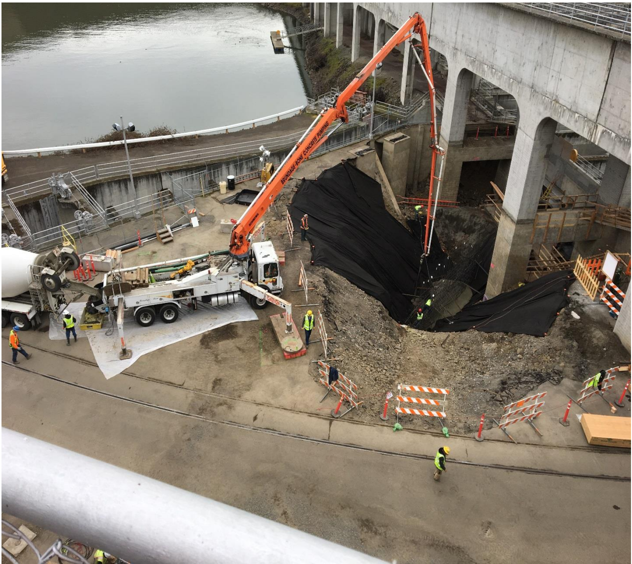
Footing poured for 7' valve room
