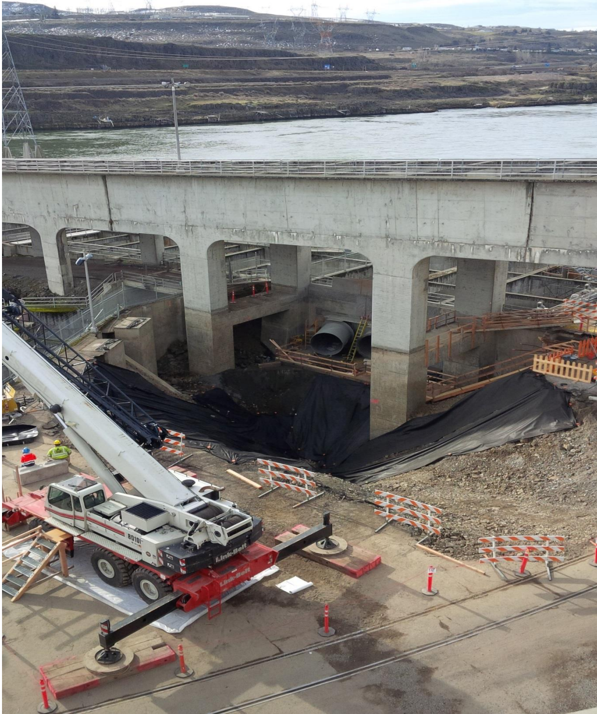
Excavation completed for 7' valve room and thrust block construction
