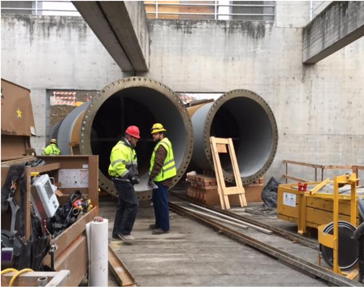
AWS 7' pipes half way across junction pool span.
