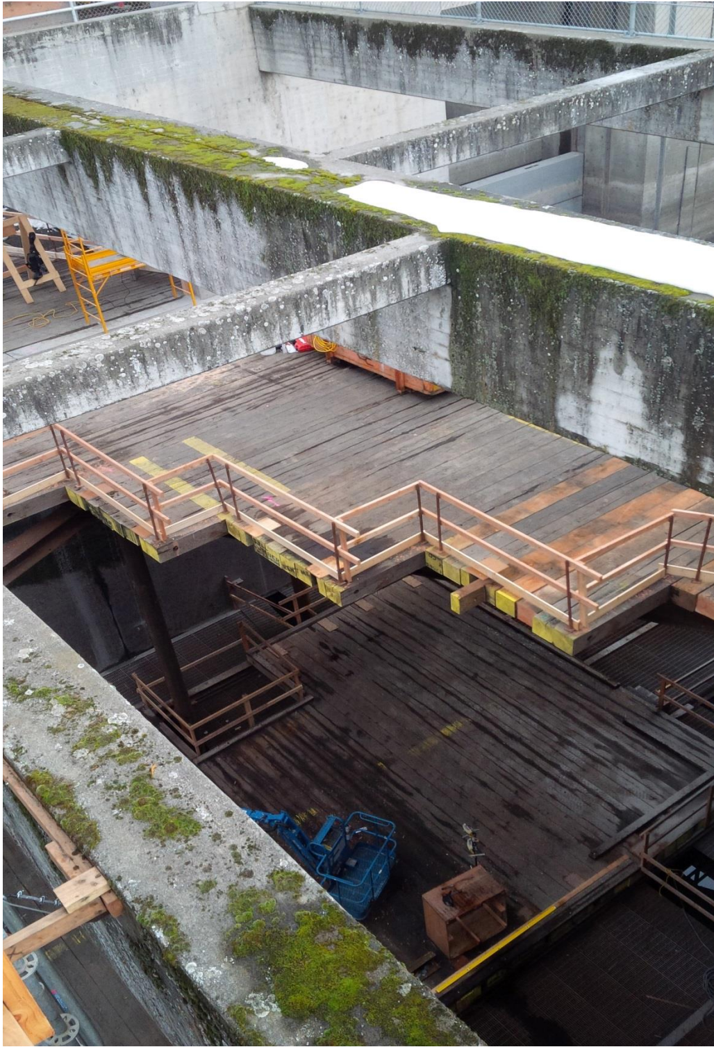
View looking into junction pool. Two levels of work platforms.
