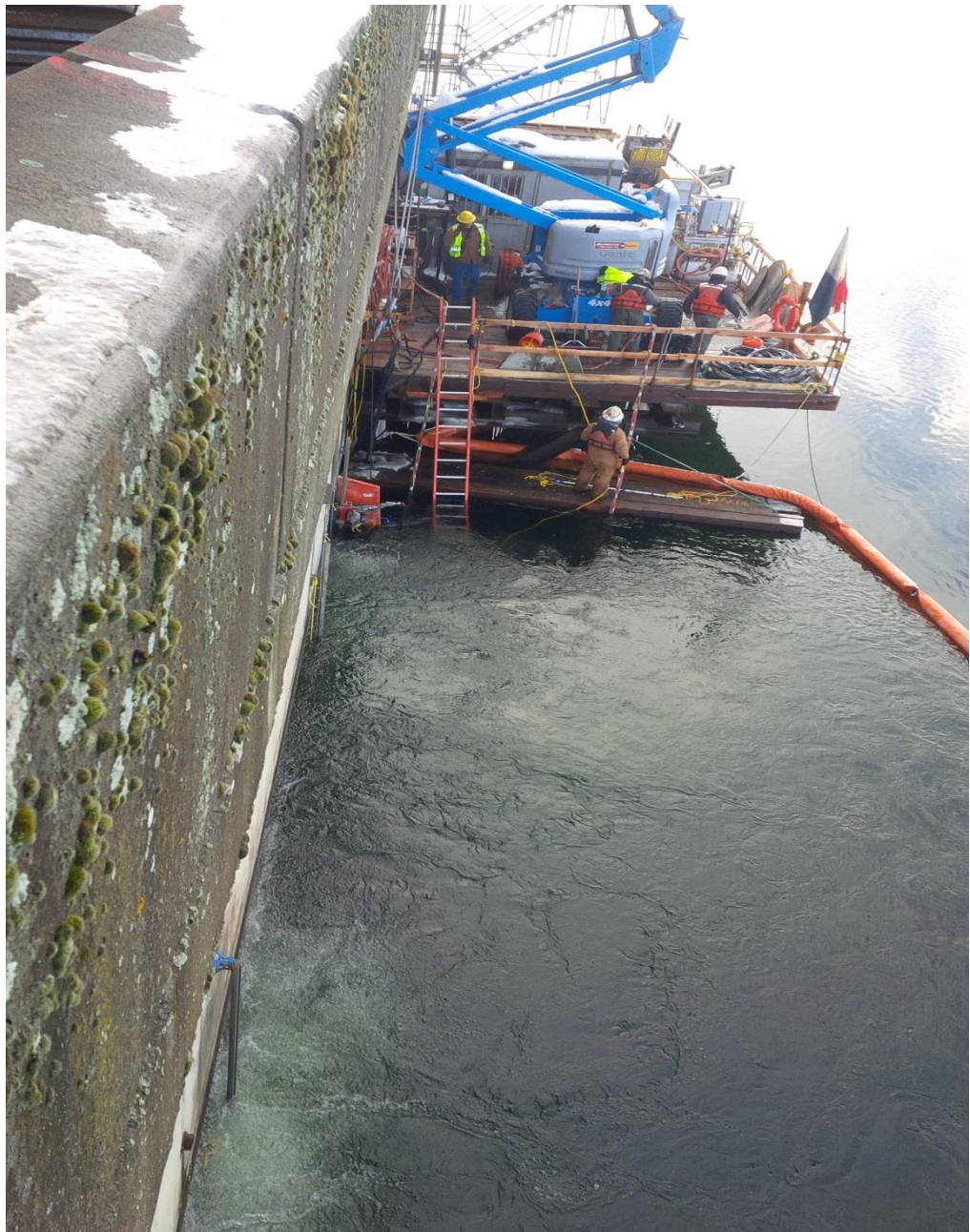
Dive operations in forebay. Slot cutting for piernose anchors.
