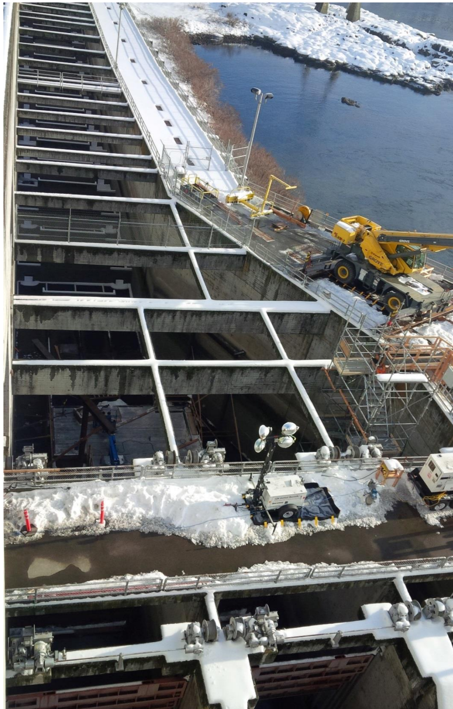
Work area in junction pool. Prep for aux water pipe crossing.
