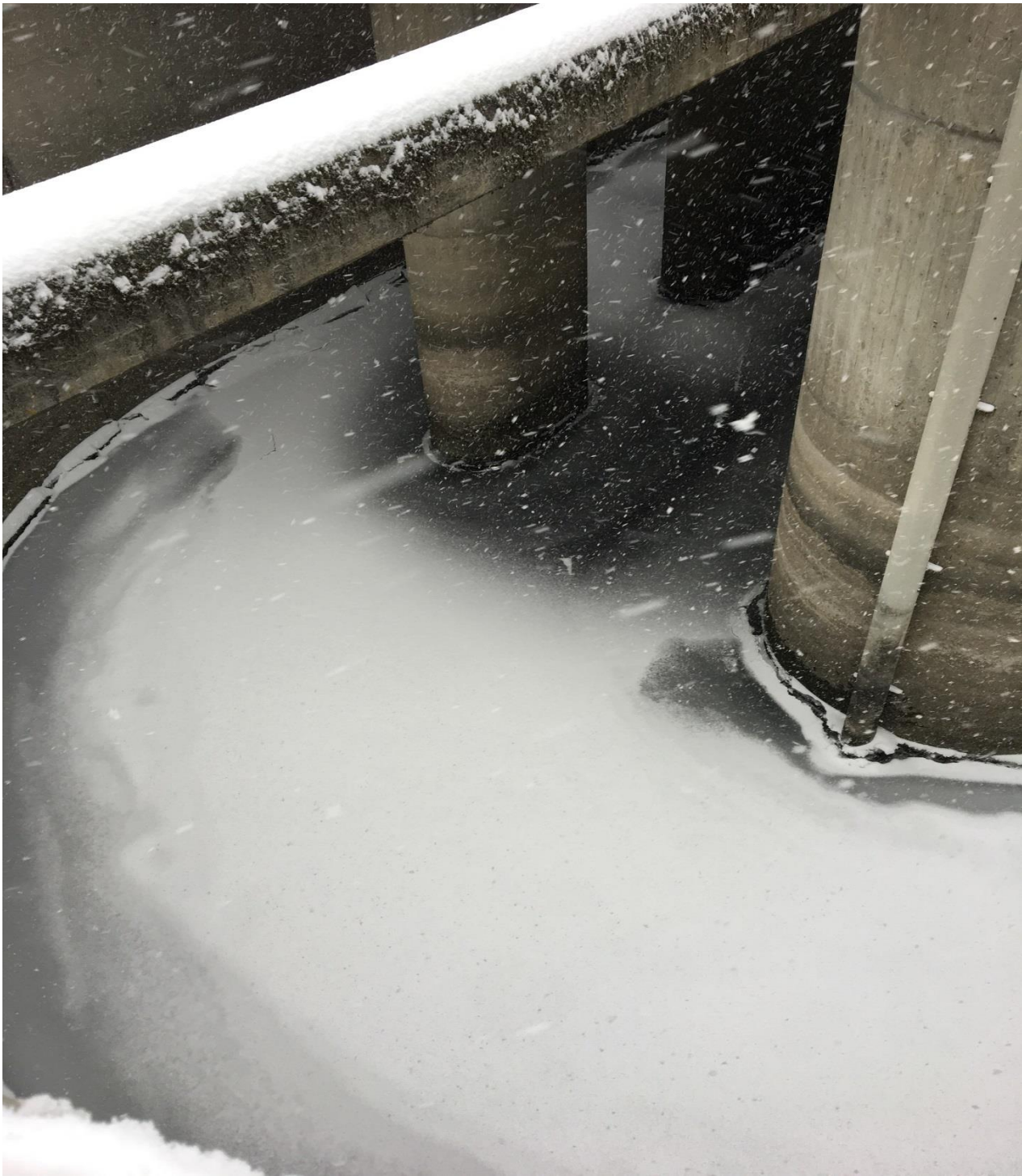
Too much ice coverage to dewater north fishway entrance below tailwater. Postponed. Would require ice fishing tactics for fish salvage.
