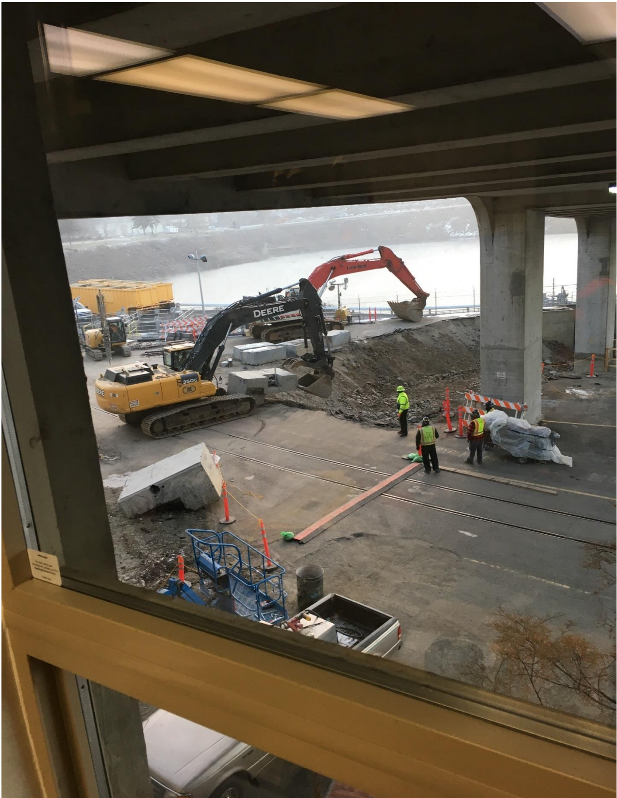
Concrete sections removed from junction pool wall
