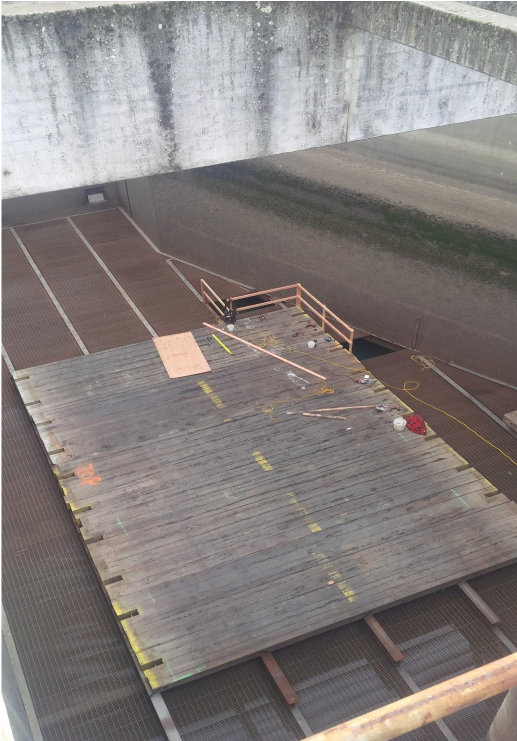
Support decking atop junction pool grating for work platform.
