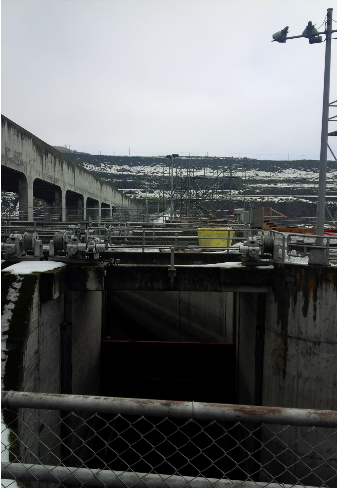
Scaffold erected for work platform installation in junction pool.
