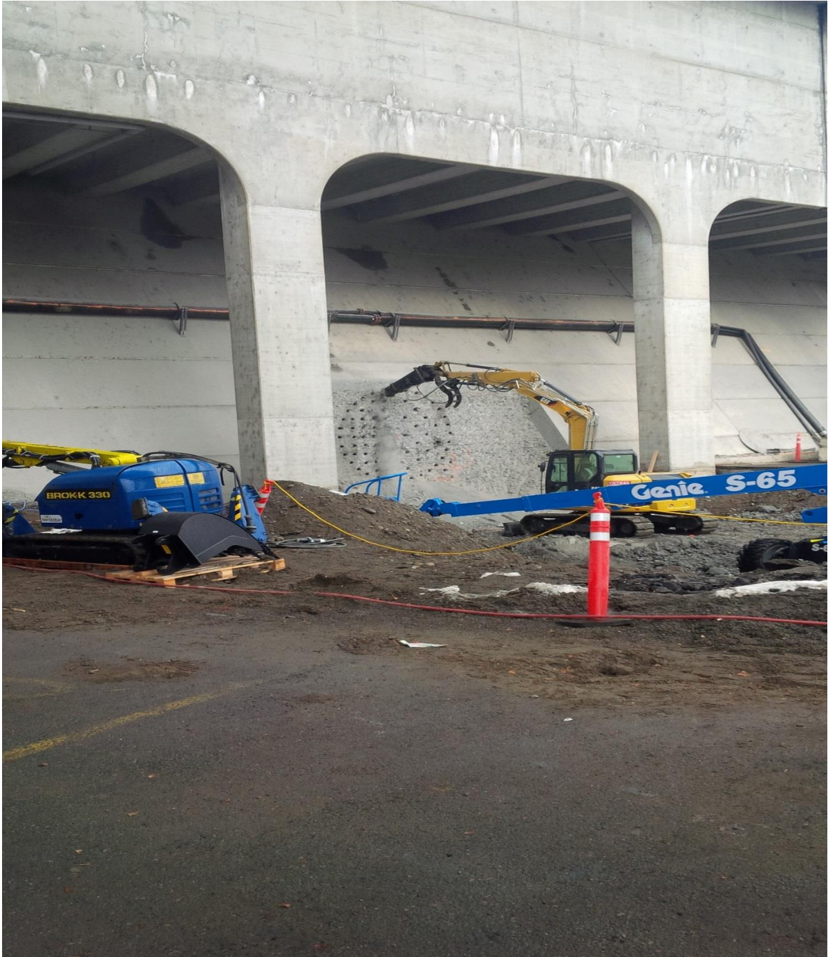
Pilot holes drilled. Jackhammering resumes.
