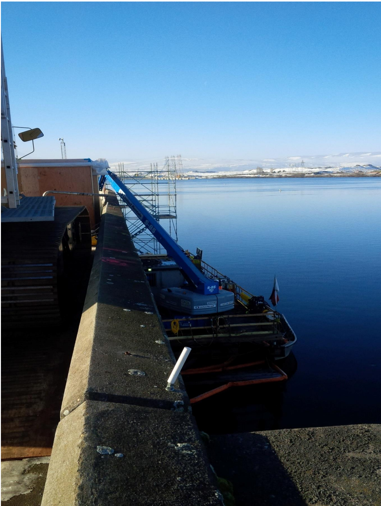
Forebay platform continues with intermittent dive work and clamshell dredging.
