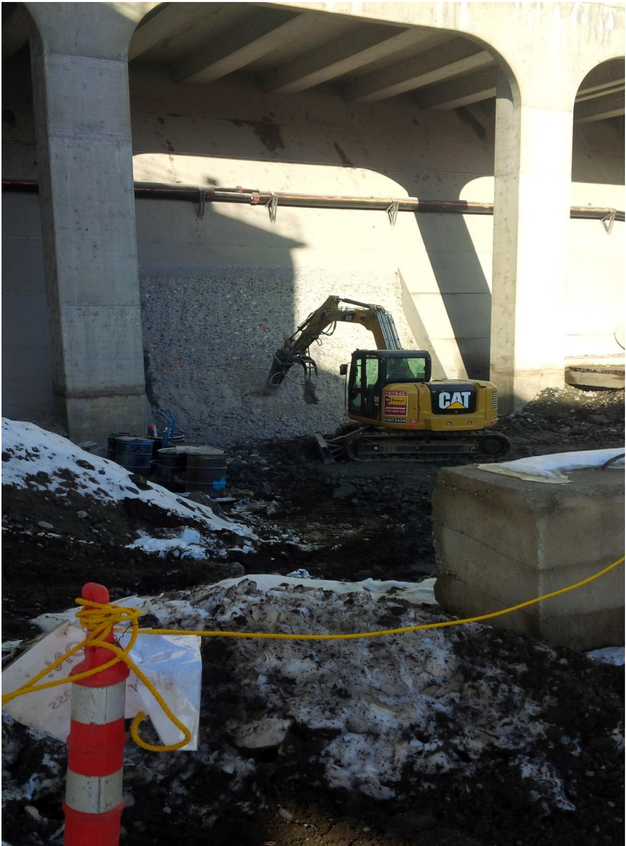
Rock hammering of dam face near complete. Prep for drilling hole.
