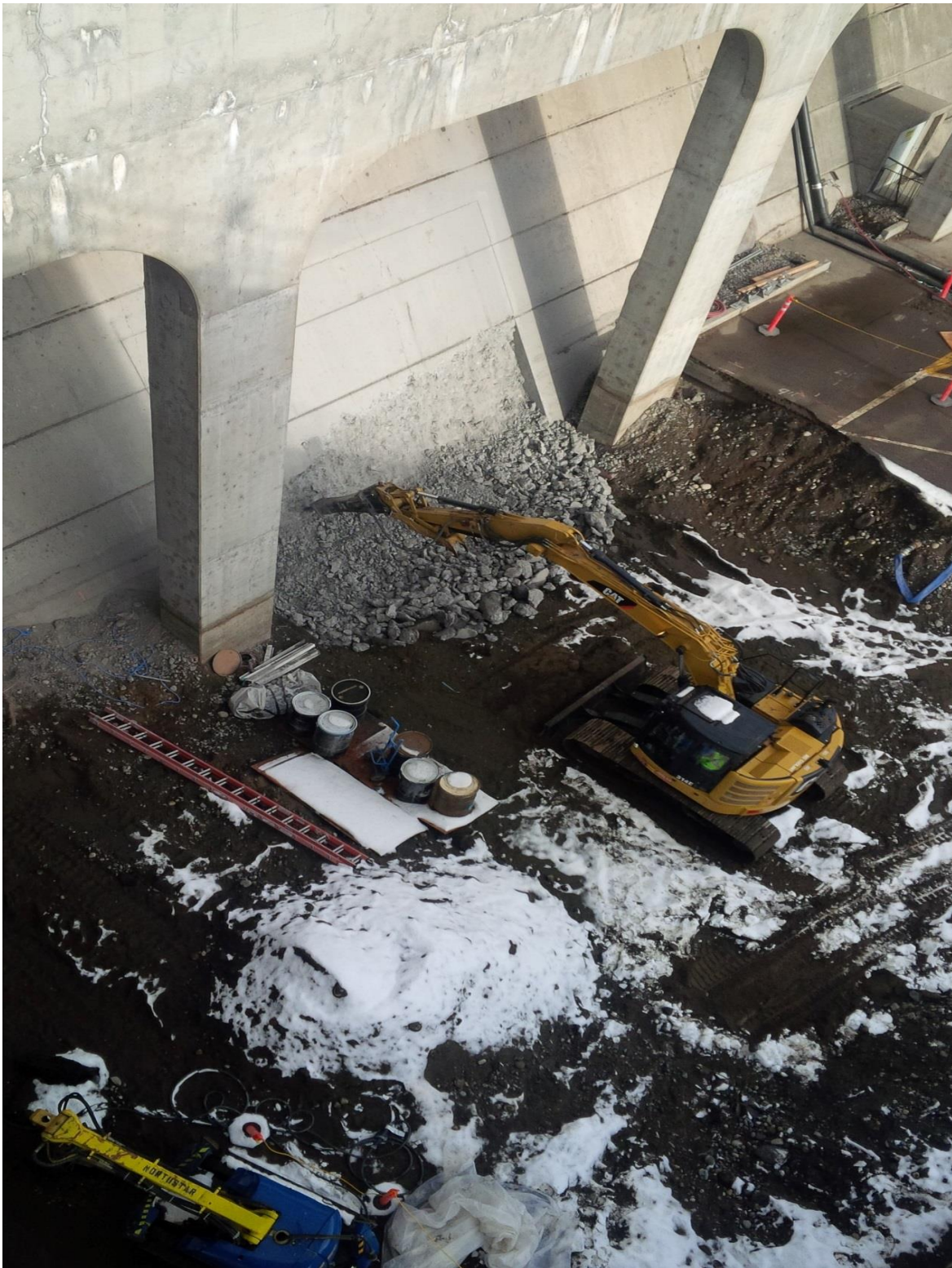
Jackhammer start on downstream dam face.
