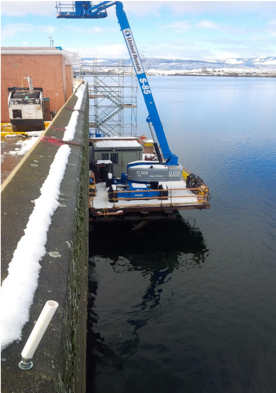
Forebay work platform
