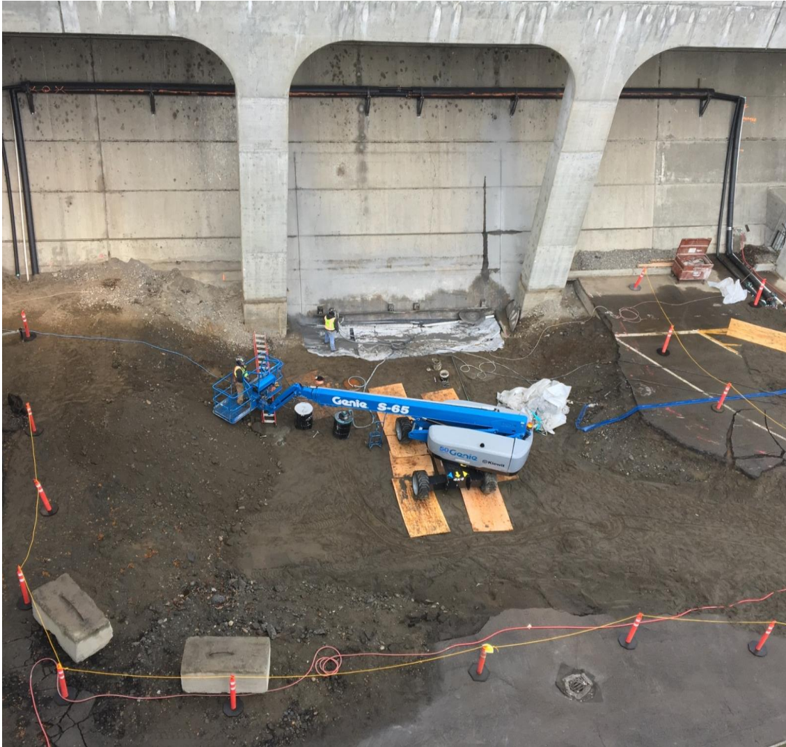
AWS backup concrete boring preparation
