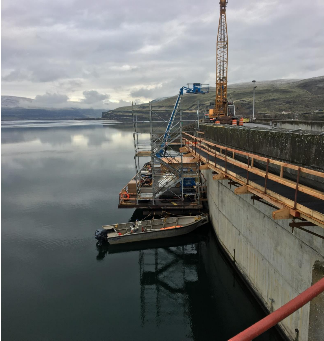
AWS backup forebay work/ dive platform
