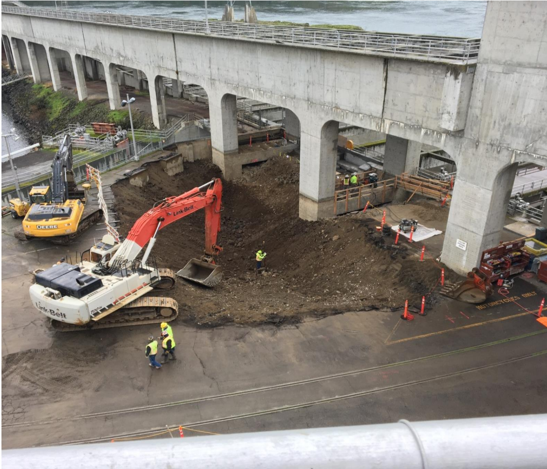
AWS backup excavation progress
