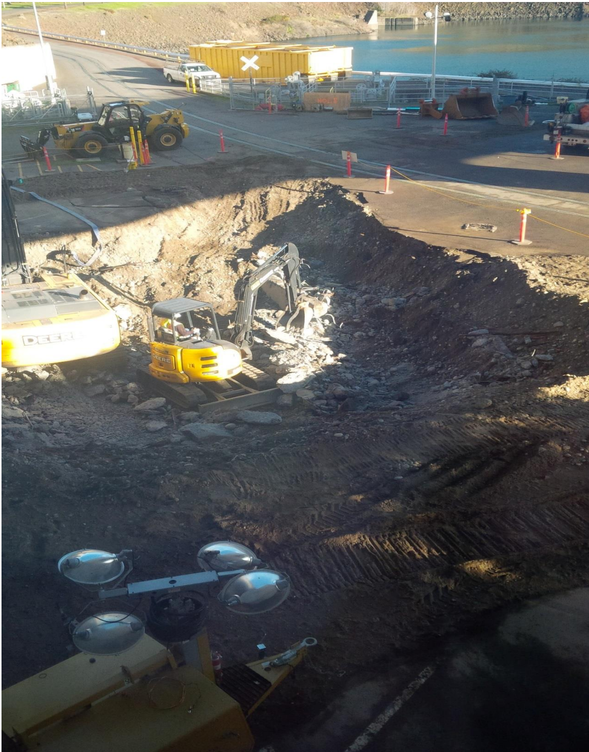
Day removal of south beam >50' from the fishladder
