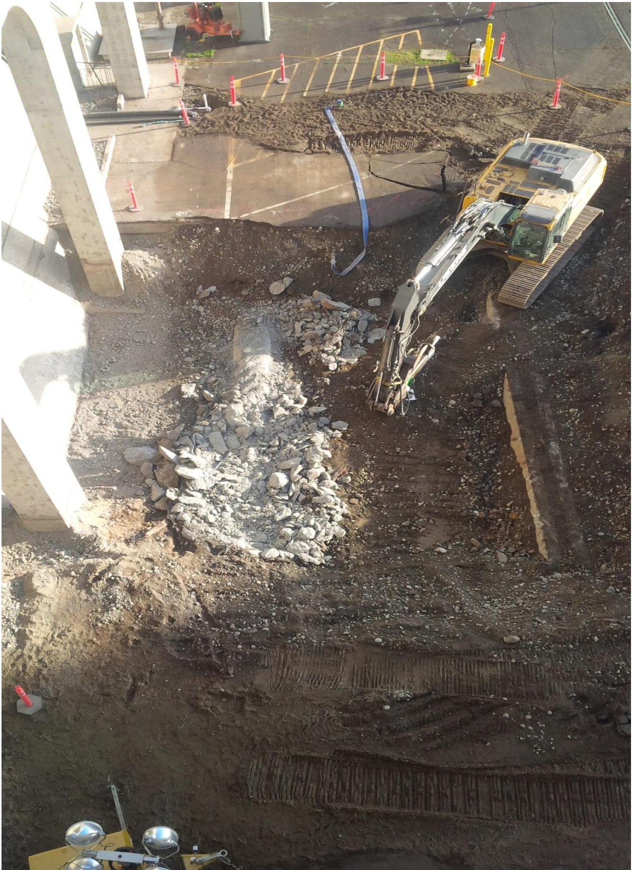
Night work progress for removal of north beam <50' from the fishladder.
