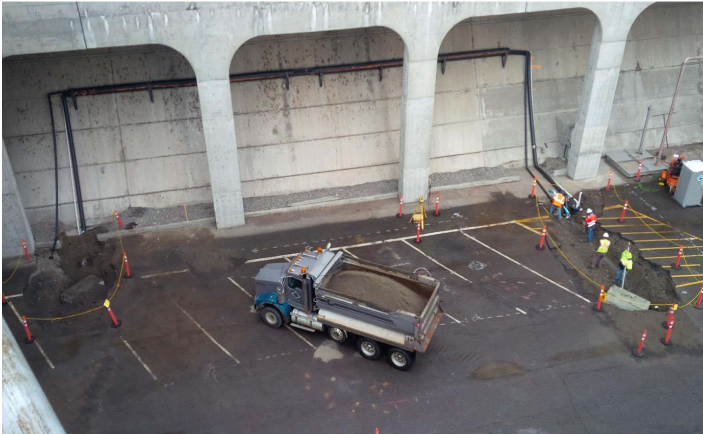
Rerouting water and sewer lines for EFL AWS 10' hole.
