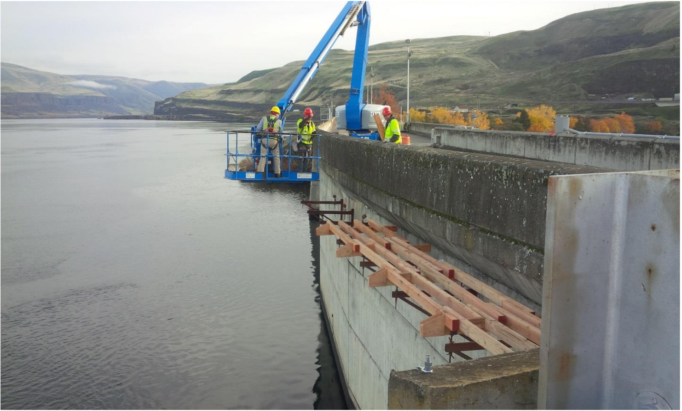
EFL AWS work on forebay side. Installing dive/work platform.
