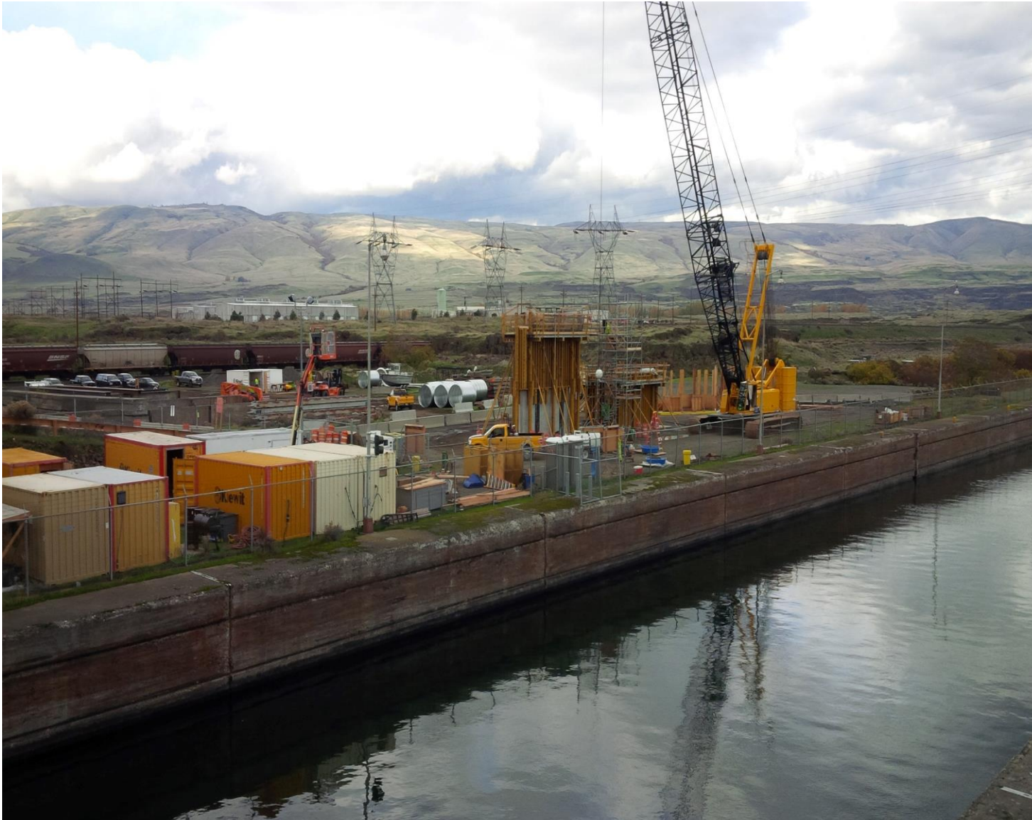
Prefab of intakes blocks continues for EFL AWS.
