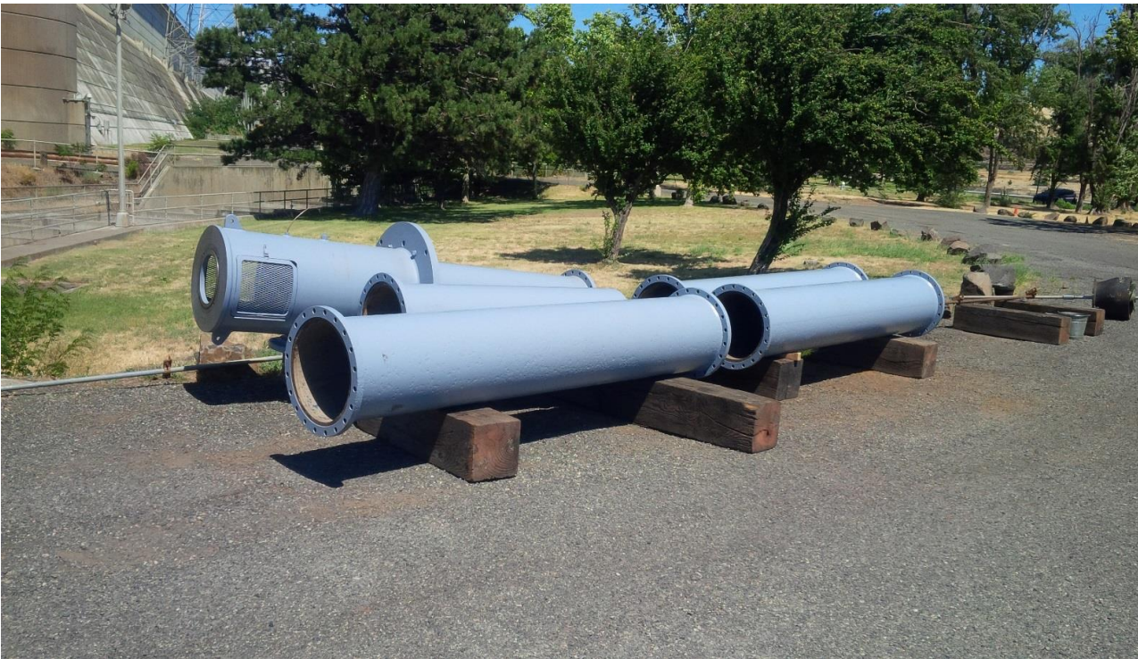
Progress on East fishway south dewater pump rehab.
