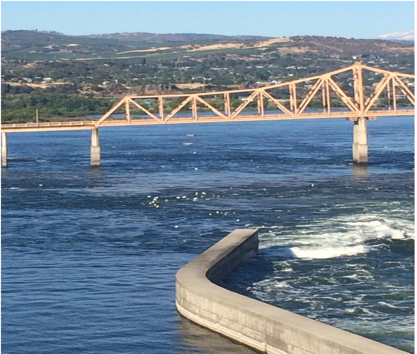
Pelicans congregating at end of spillwall. They access flying under bridge and avian lines.
