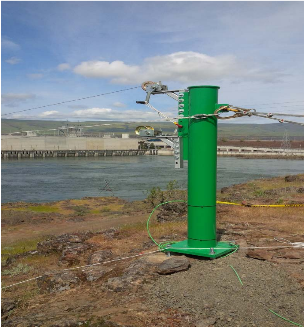
New avian line pole for west powerhouse. 18 of 26 lines recovered from failure
