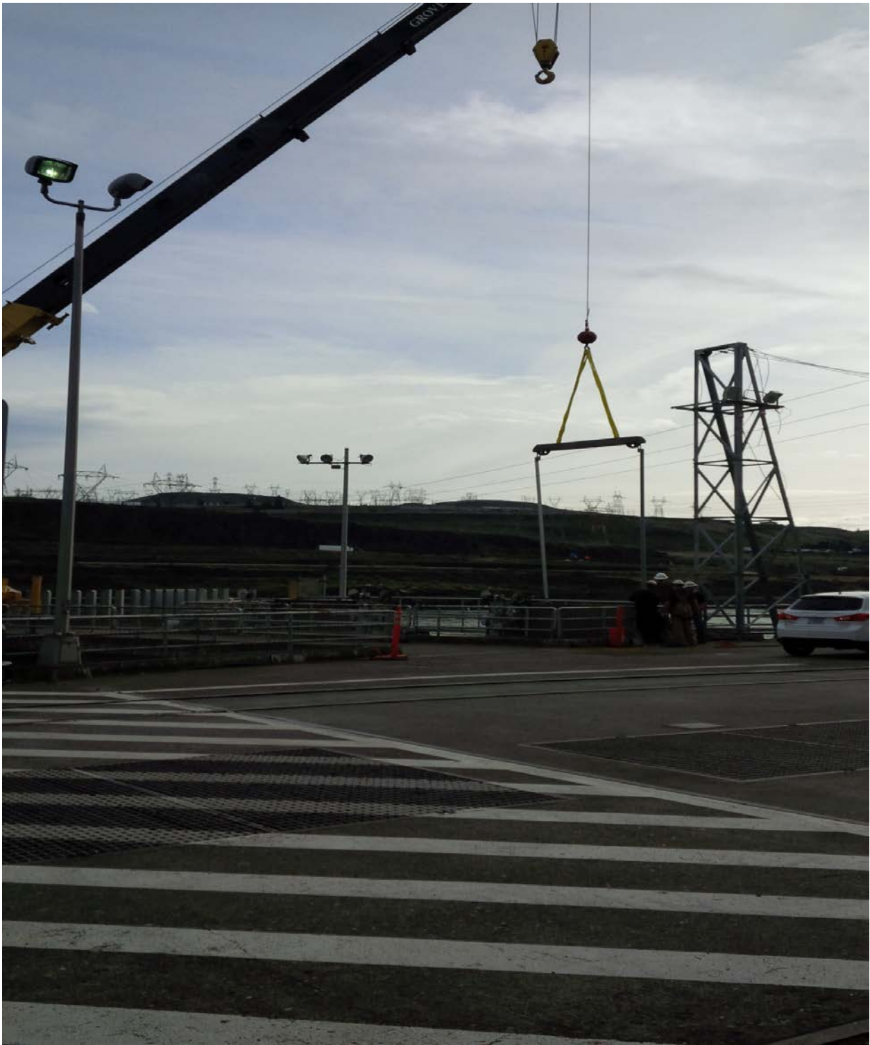
Installation of east entrance modified weirs and weir extensions.
