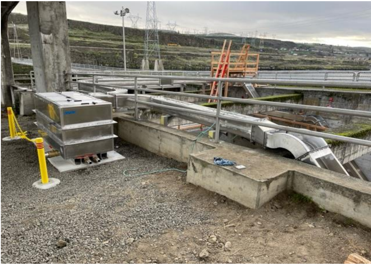
LPS almost ready for water. 1.4.24
