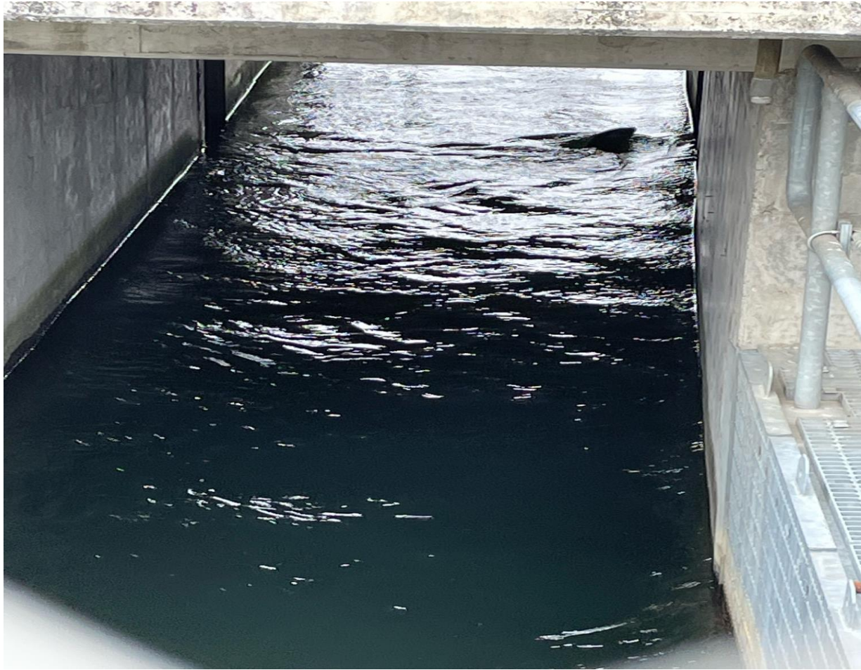
River otter observed in north fishladder. Attempting to trap.
