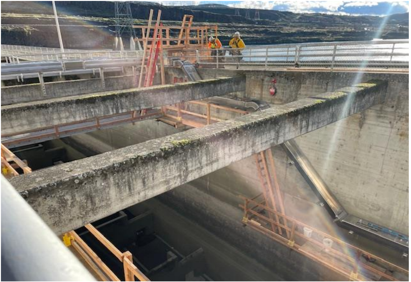
Contractor work on the Lamprey Passage System continues 12/21/23
