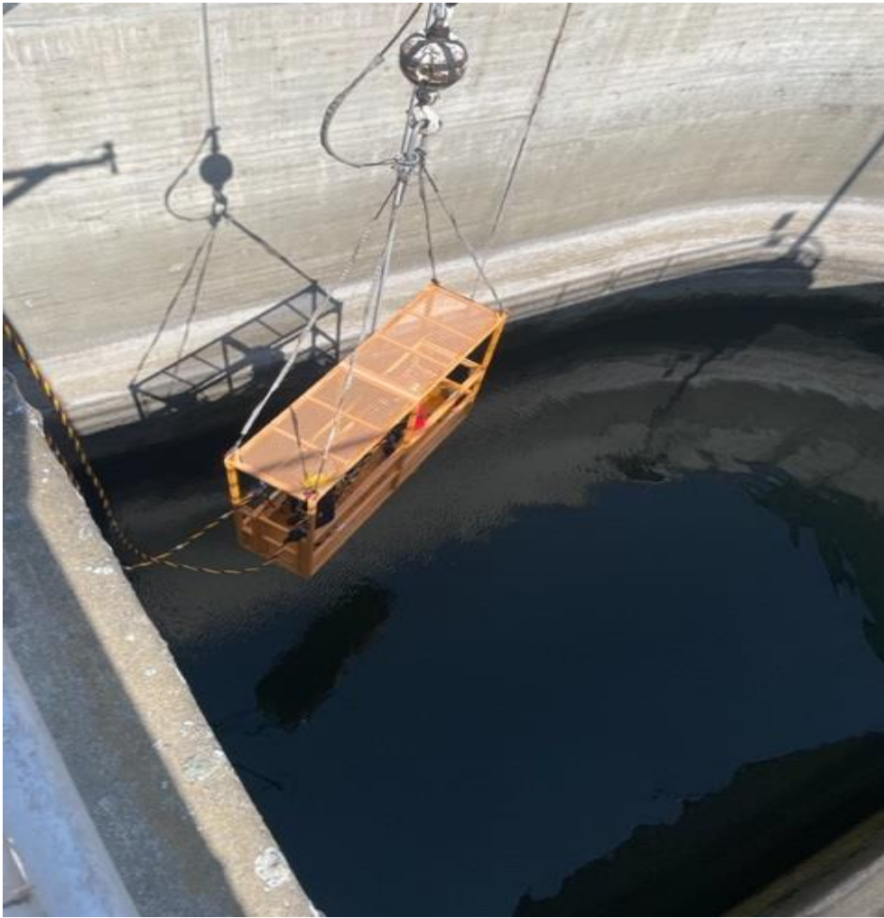
Grating repair dive Aug16
