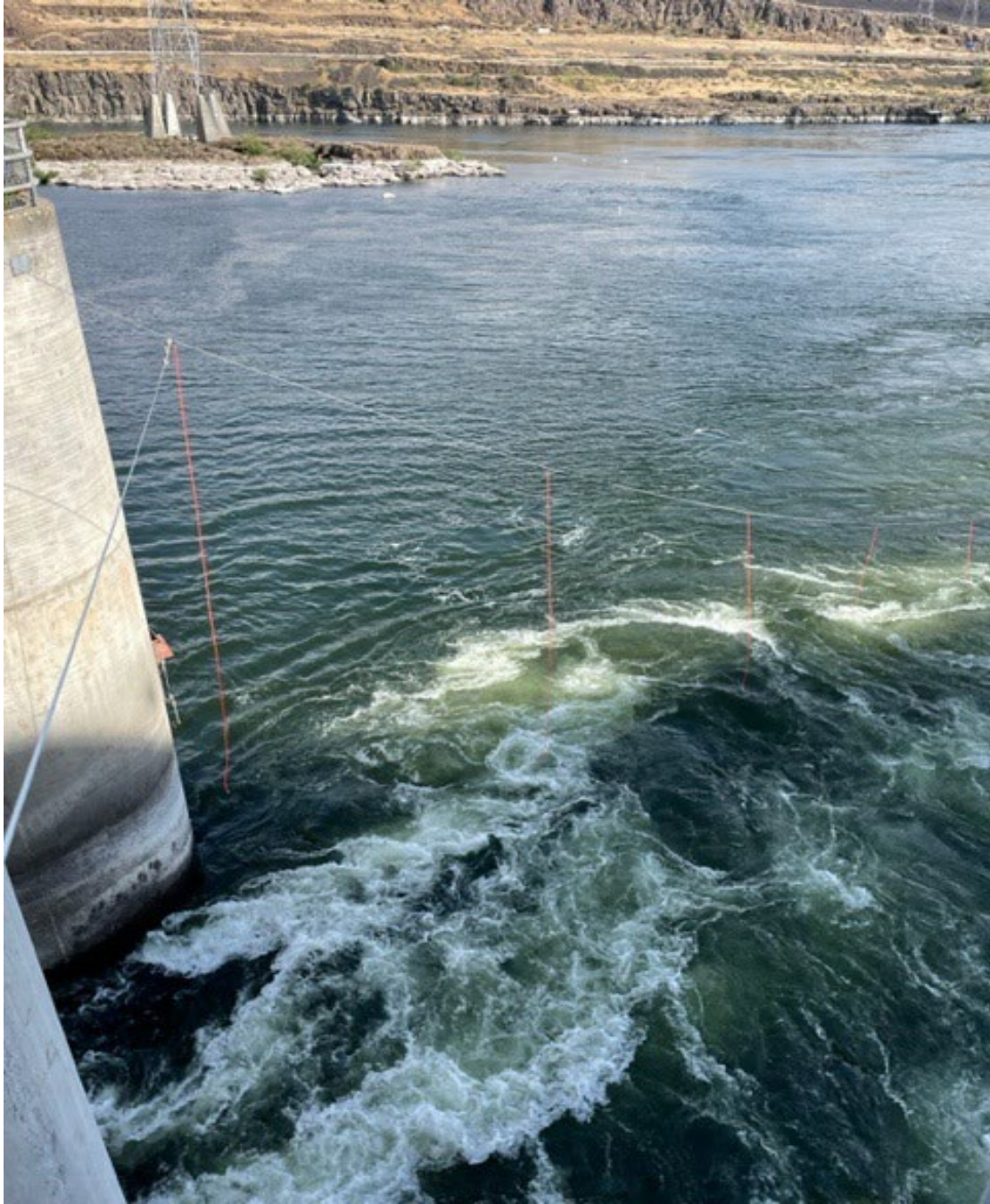
Tori line first deployed 6/28. Pelicans are backing off.
