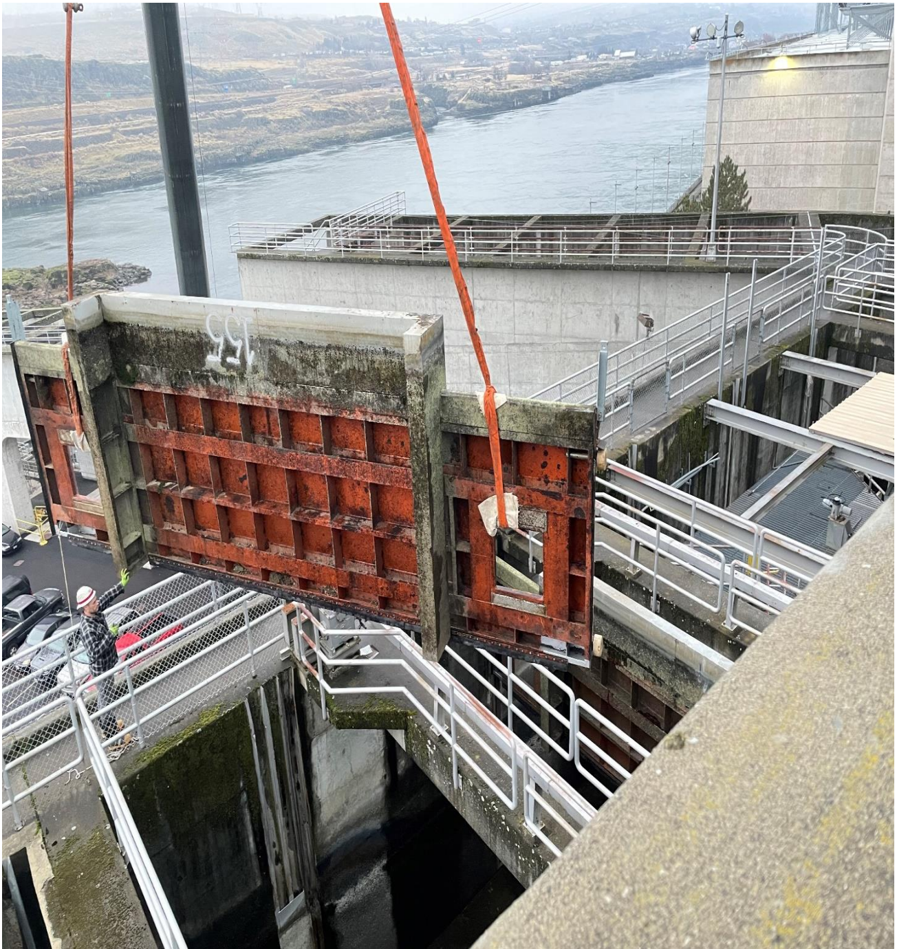
Repaired 155 weir installation. Lamprey orifices cut in bottom corners.
