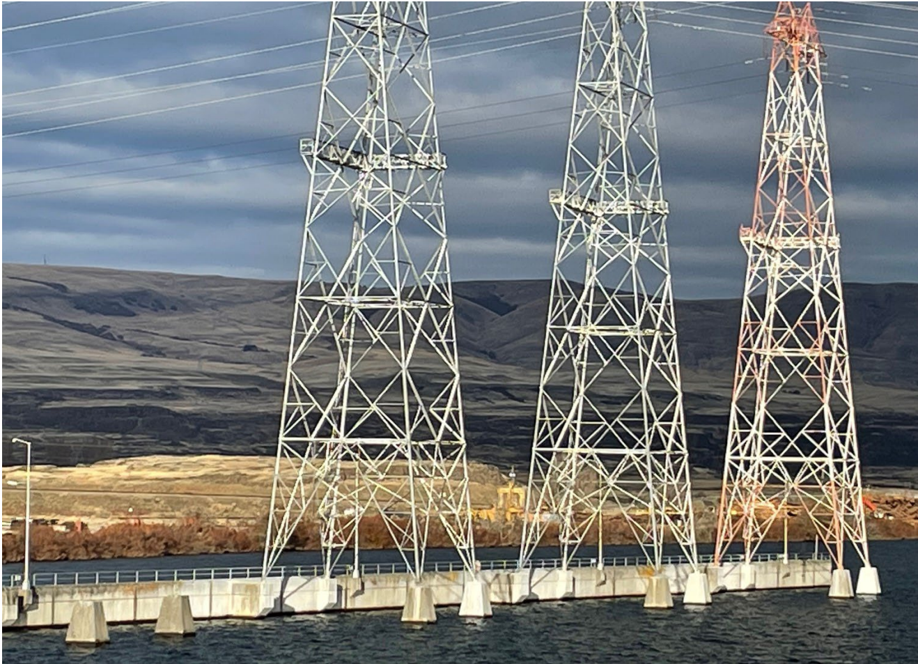
BPA towers show white staining at bases from cormorant droppings 12/2 Dead cormorant, not seen in picture, hanging from middle tower, caught in fishing line??
