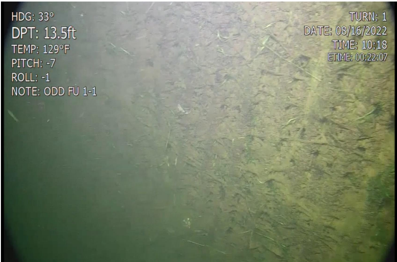
Fish unit trashrack inspection
