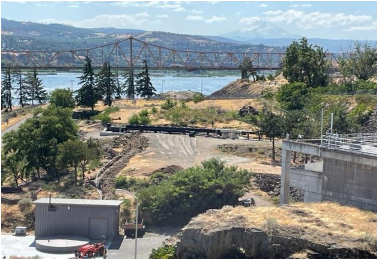
Progress being made on North PUD sampling facility.
