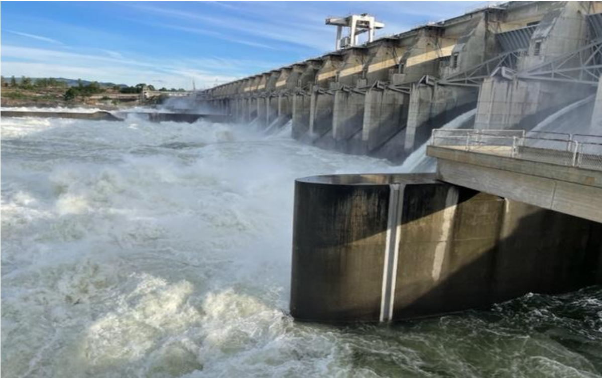
Spilling south of spillwall.
