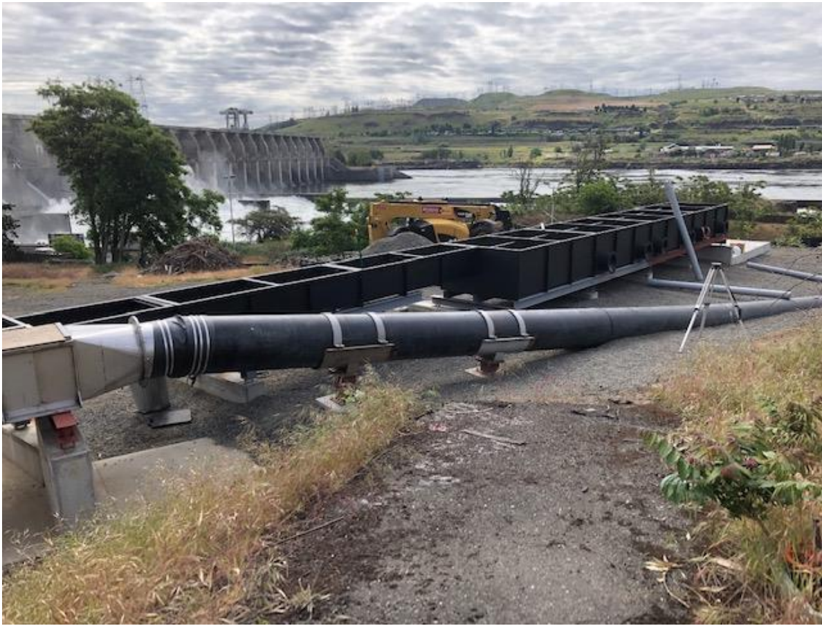
Progress on PUD sample facility construction
