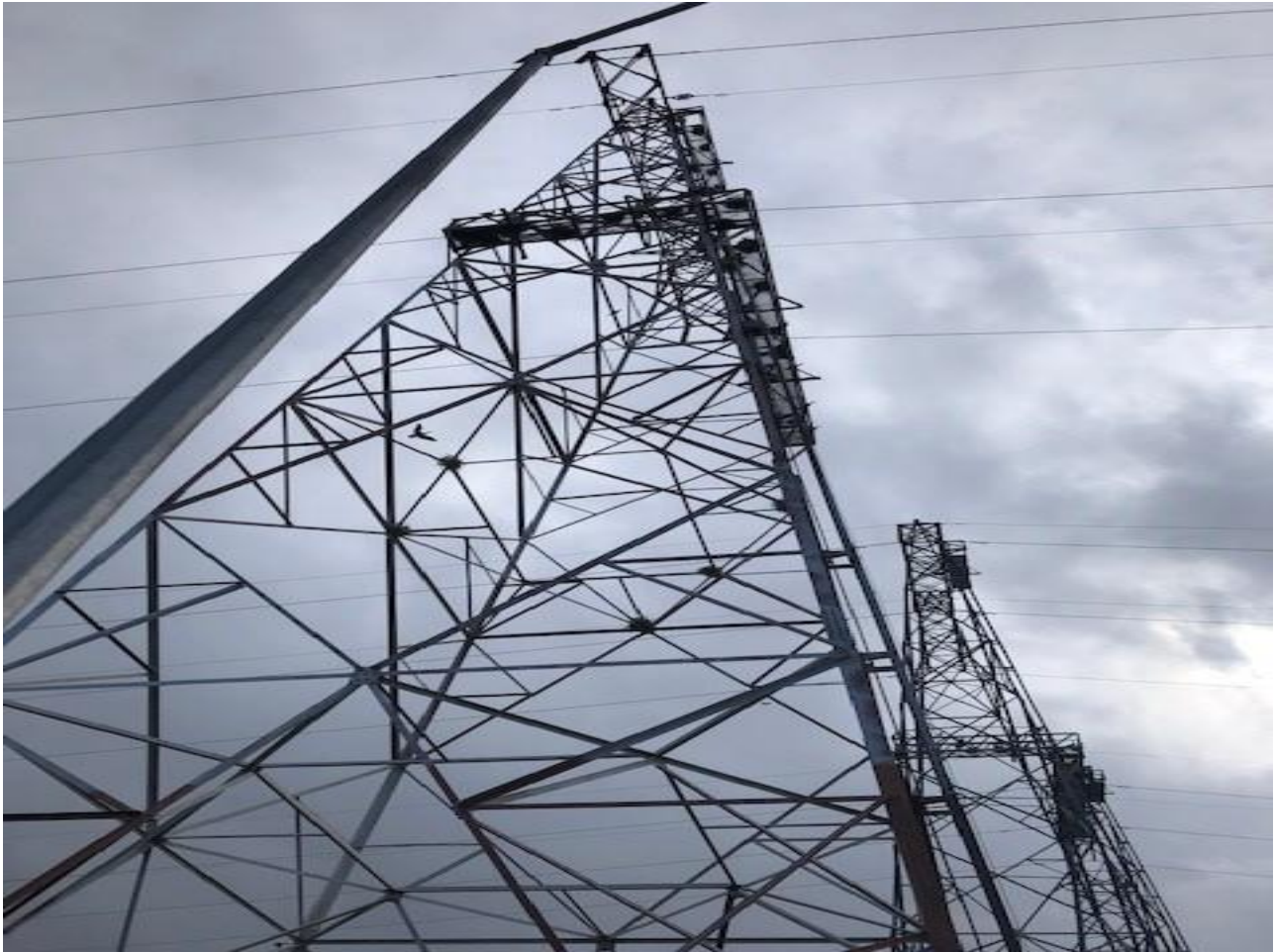
Cormorant nests in forebay towers. Numerous PITs scanned below.
