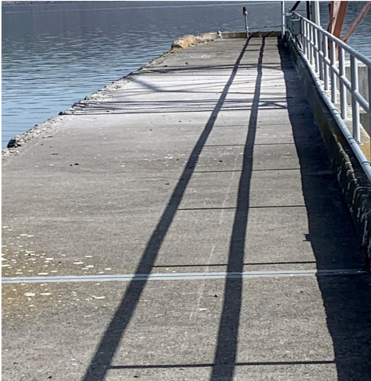
Upstream Navlock guidewall PIT scanned.
