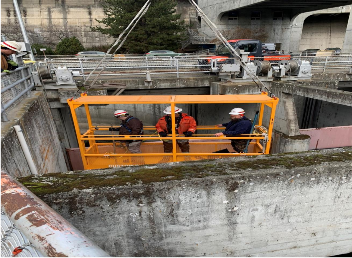
Dewater lower channel 12/8/2021
