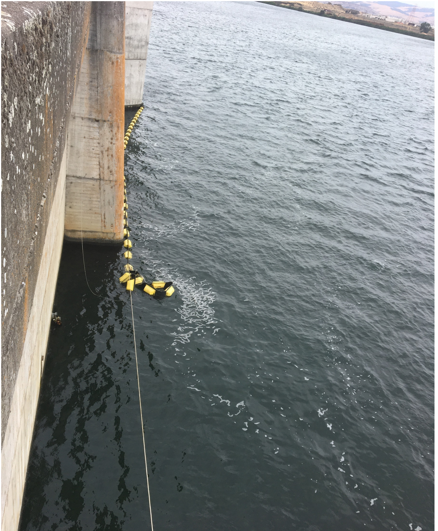
current-temporary status east exit oil boom
