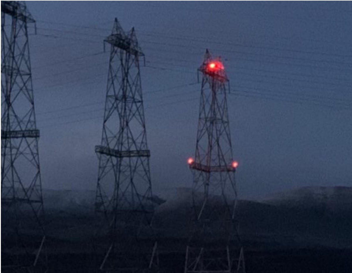
Laser most effective during twilight to deter comorants from overnight roosting. Detering up to 135 cormorants.
