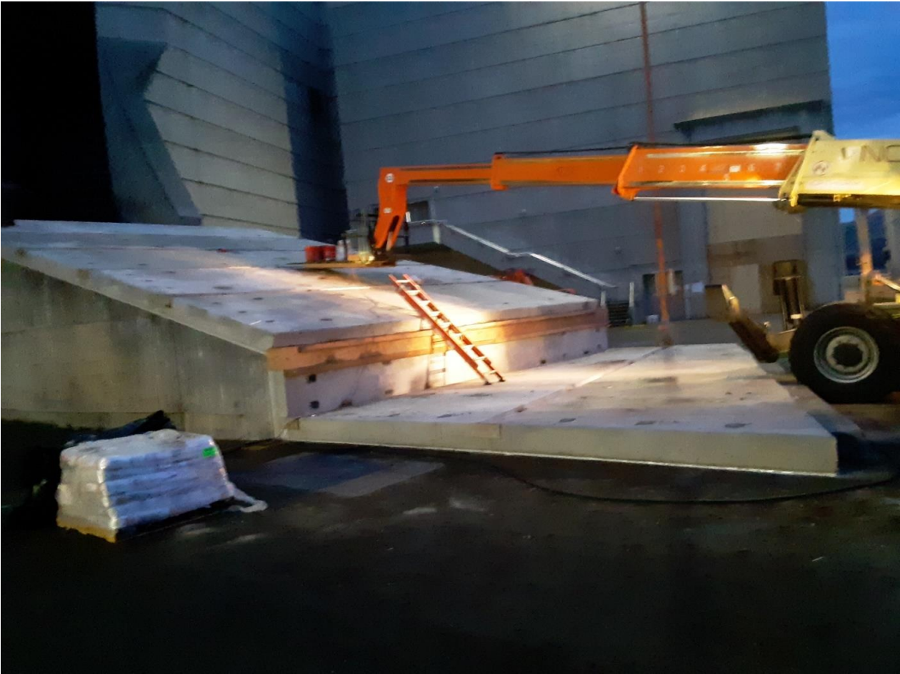
New sluiceway cover to prevent spray and icing
