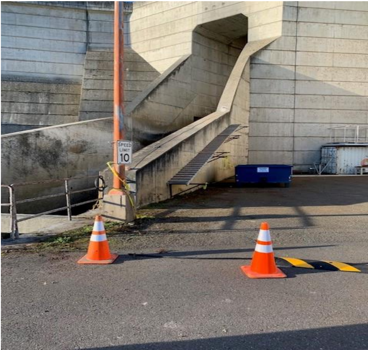
Contractor preparing work site for sluiceway cover
