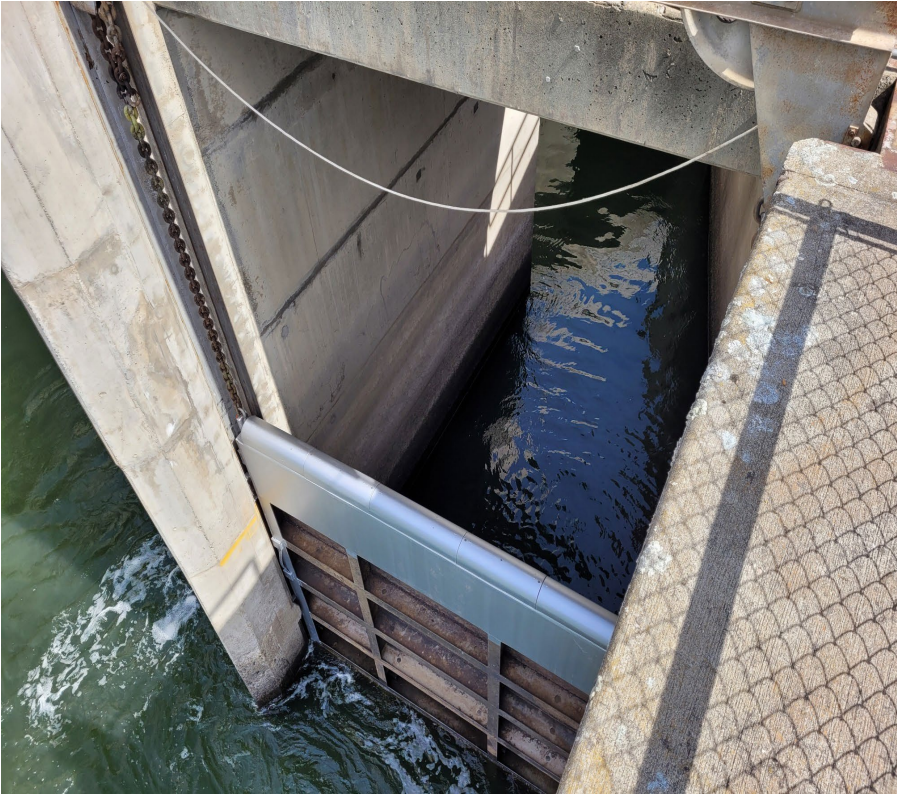
New SE1 entrance weir with front plate and rounded top installed 04/23/24
