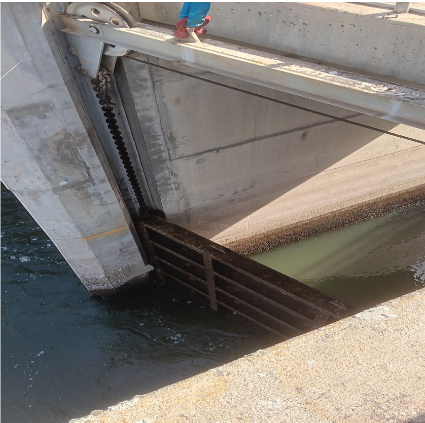
Previous SE1 entrance weir removed
