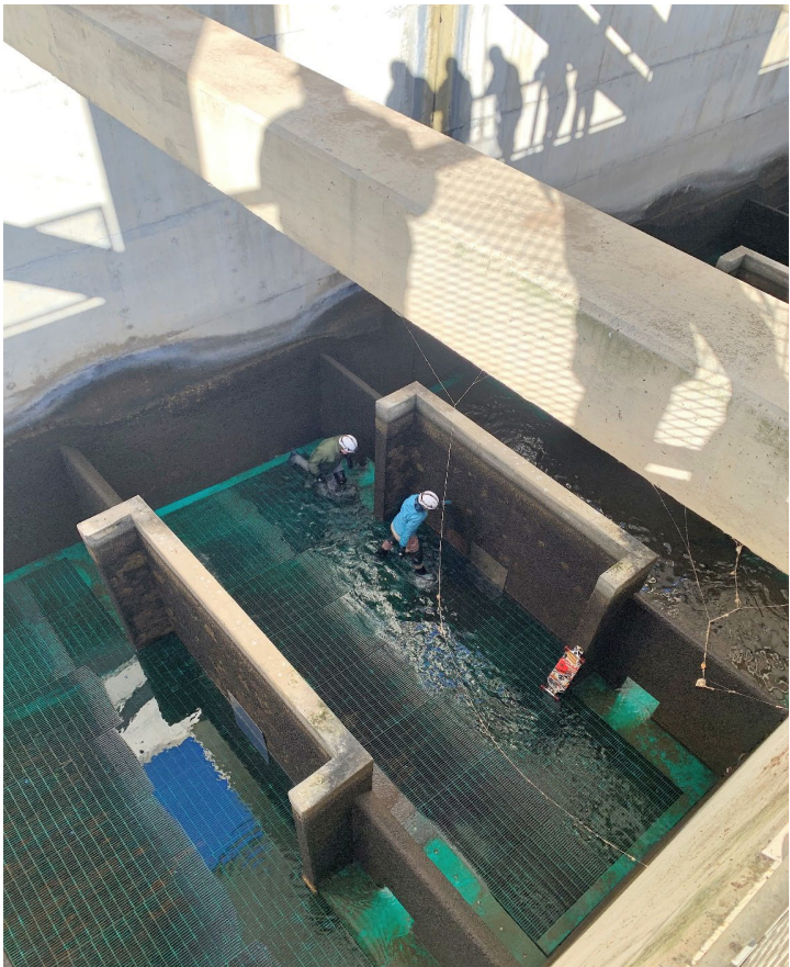
NFL dewater fish salvage (12/1/22)
