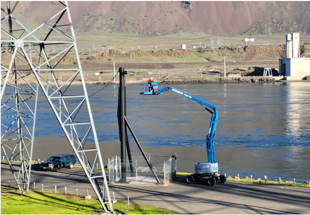
Avian Line Repair Completed 3/29/22
