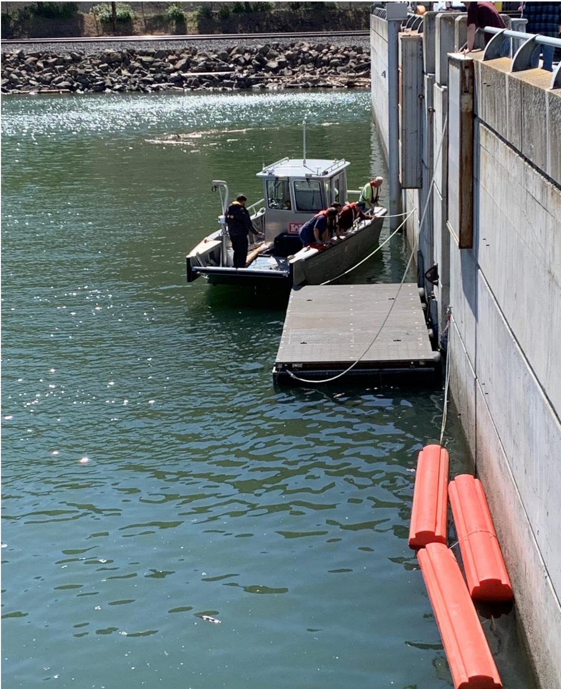
Temporary boom installed at south fish ladder exit. Boom was installed 5/4/21
