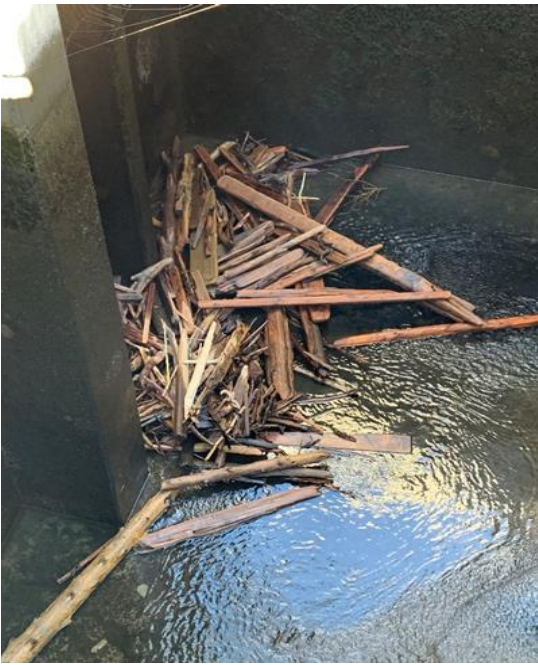
Debris mat in SFL
