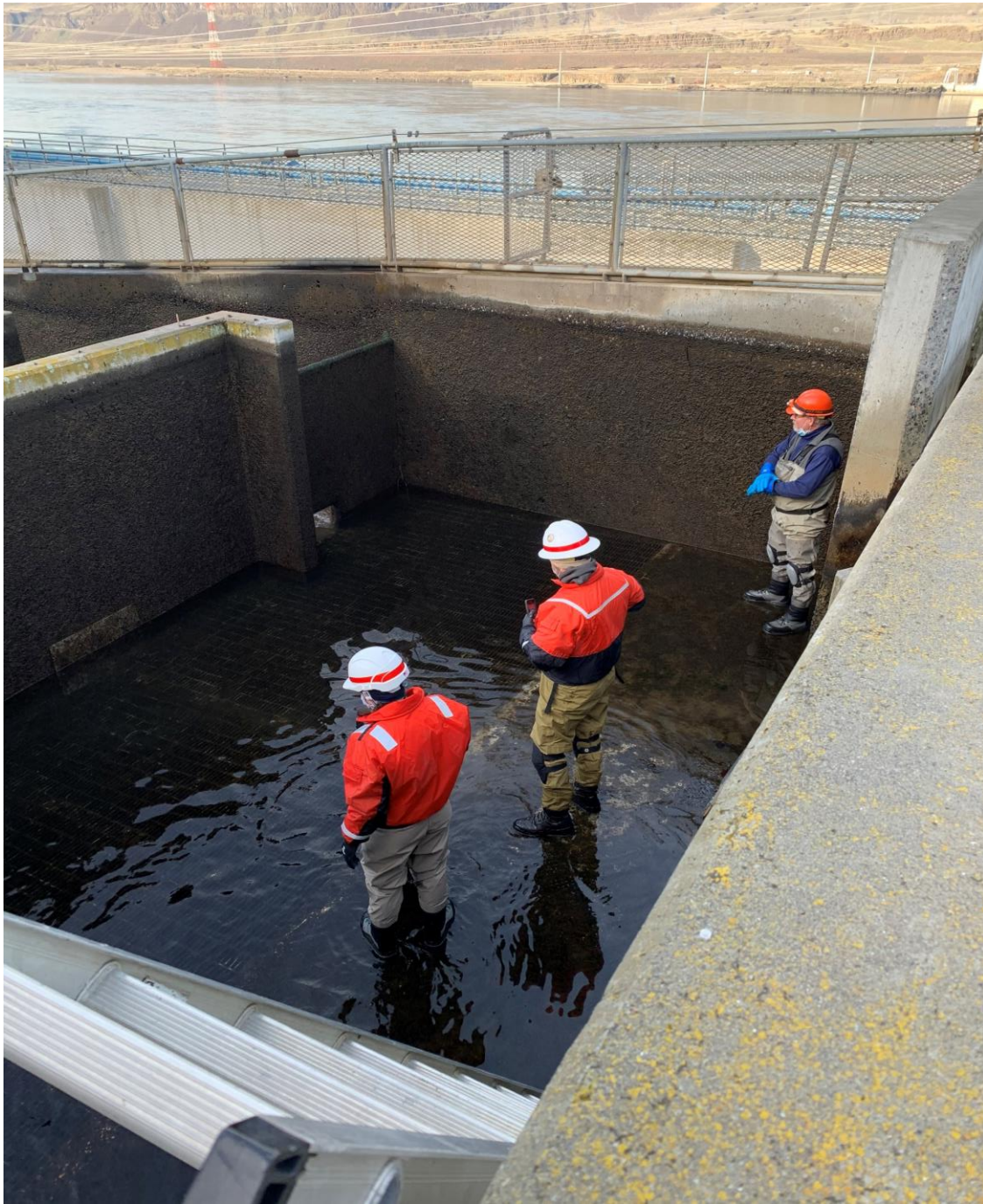
South fish ladder dewatering 19 January.
