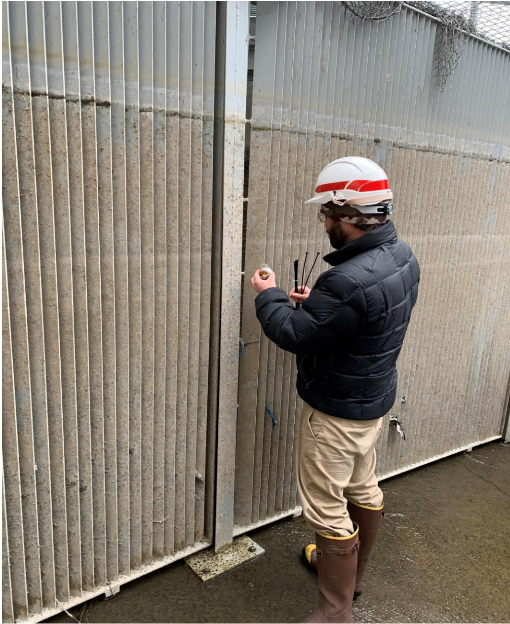
Installing a HOBO Temperature Probe in the North Fish Ladder
