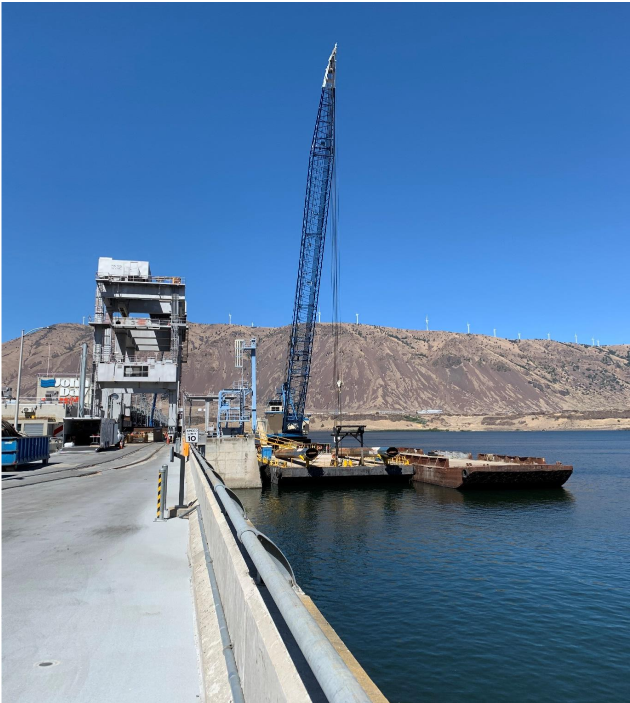
Intake crane demolition
