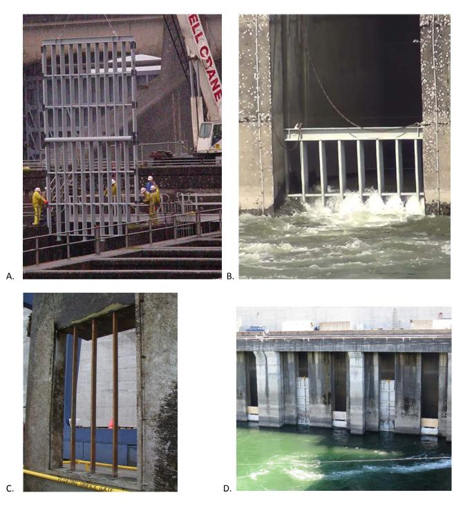
Figure 14. Sea lion exclusion device (SLED) at Bonneville Dam fishway entrance (A) (Tackley et al. 2008) and installed (B) (photo by Bjorn van der Leeuw, USACE FFU), floating orifice gate (FOG) (C) (unknown source), and sea lion incursion barriers on top of FOGs (D) (photo by Patricia Madson, USACE FFU).
